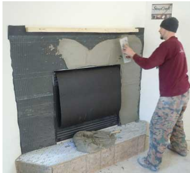
Setting bed being applied directly to scratch coat.
