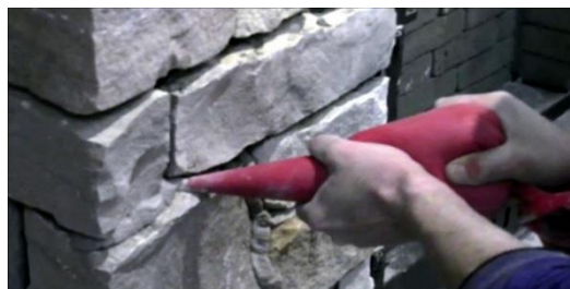
Above: Example of joint grouting.
