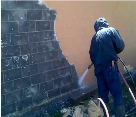
Sandblasting CMU wall to remove non-cementitious material.
