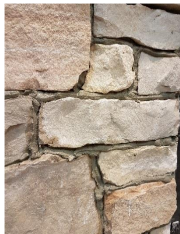
Below: Example of finished grouting.
