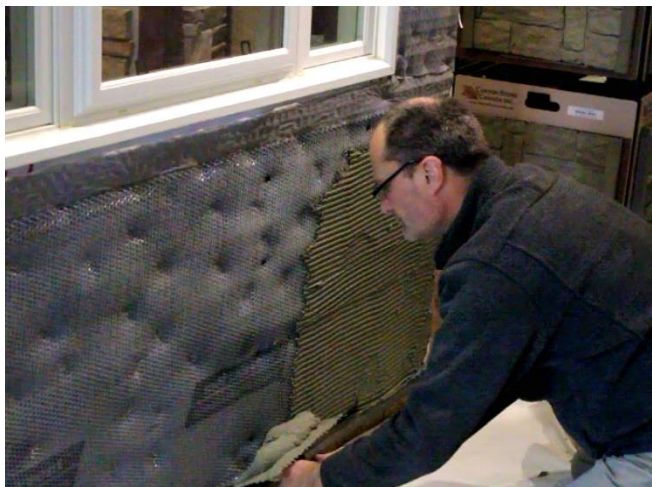
Scratch coat being applied to metal lath.
