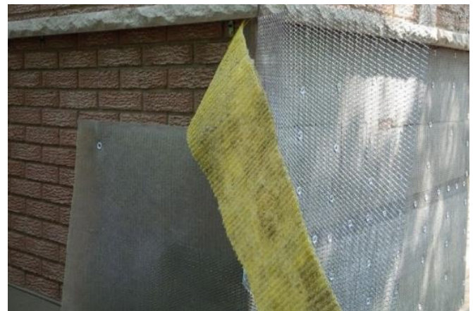
Metal lath attached to exterior brick veneer.
