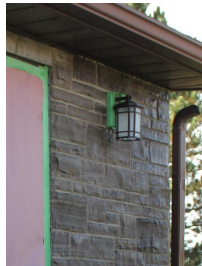
Example of applying sealer.
