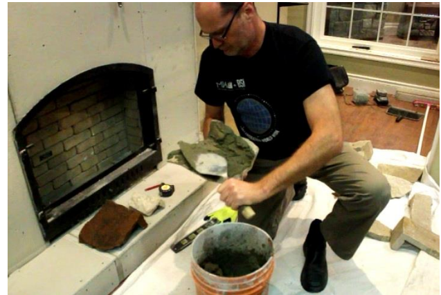
Above and below, examples of applying mortar directly to back of stone. Also referred to as "buttering" back of stone.
