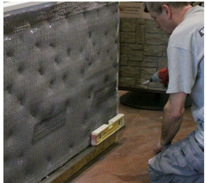
Metal lath being fastened to wall
