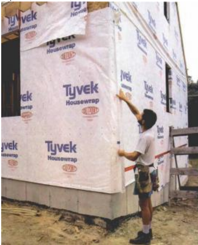
WRB being installed to structure.
