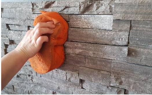
Washing stone with damp sponge prior to finishing.
