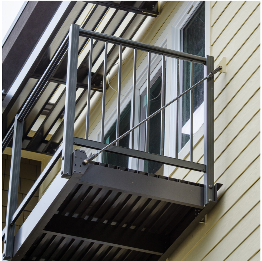
Figure 6. This lightweight, prefabricated aluminum balcony is designed with integral diagonal support rods that connect to brackets that are through-bolted to the house framing.
