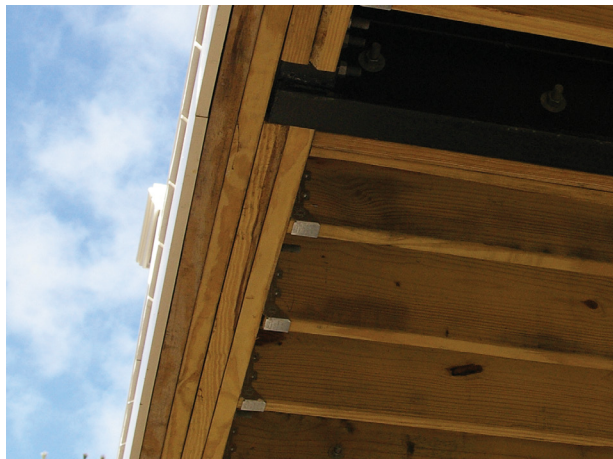
Figure 4. Pressure-treated 2x12s were used for the perimeter and infill joists, as well as for the ledger bolted to the house's rim joist. Adjacent joists and the rim beam were bolted to the steel.
