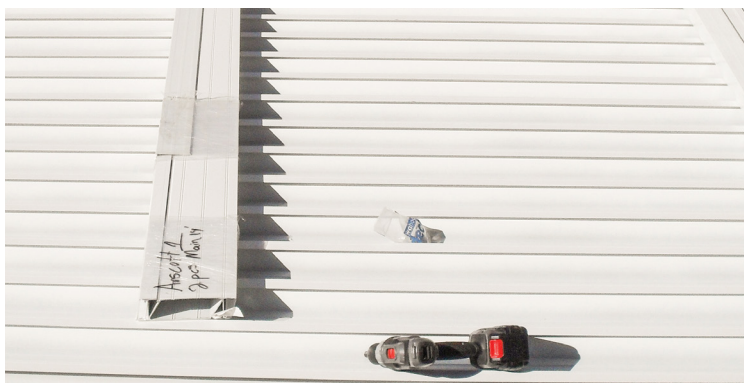
Figure 8. Wahoo Deck’s Dry Joist EZ is a 2-inch-high aluminum joist with an interlocking design that makes it waterproof. The system can span up to 8 feet, depending on floor loads.
