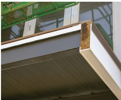
Figure 9. Any standard decking can be attached to the aluminum joists; any water that makes its way into the deck’s interior drains to the outer edge.
