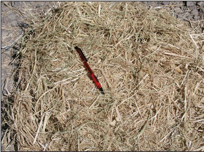
Figure 7a—Close-up of straw mulch descending fillslope with vegetation starting.
