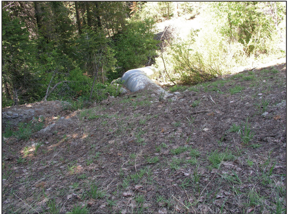
Figure 8b—Sprayed mulch on descending fillslope with vegetation starting.
