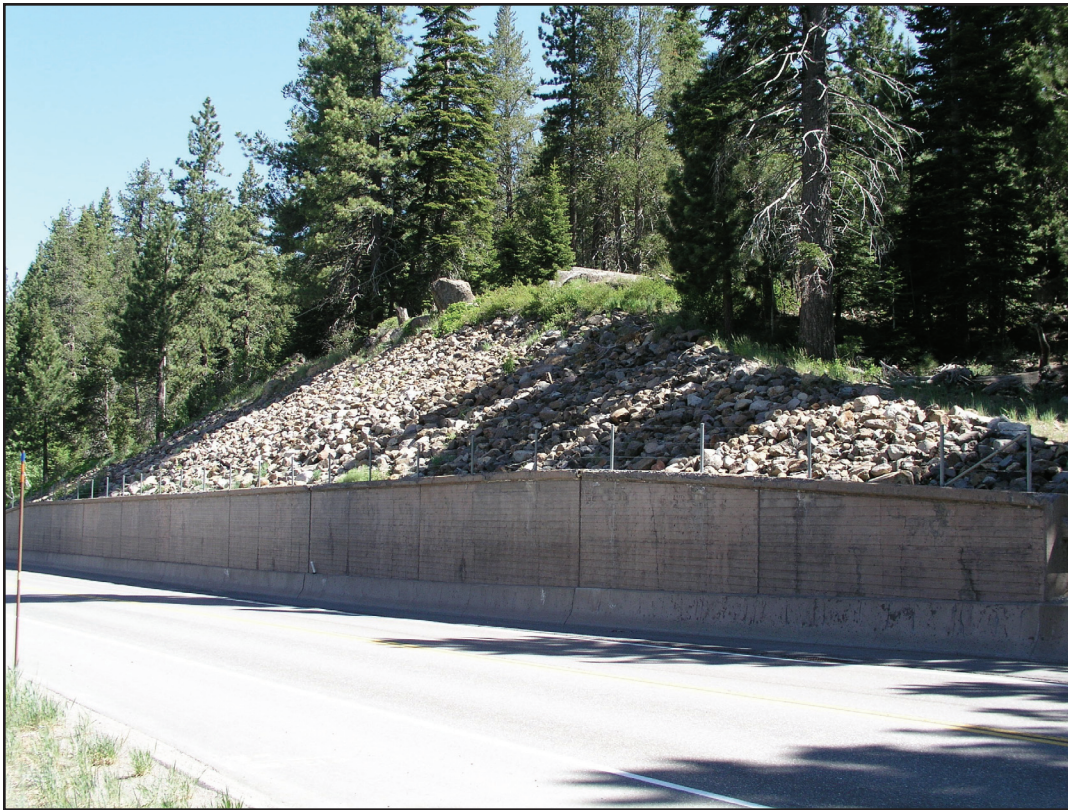
Figure 12—Riprap erosion protection on cutslope above retaining wall.
