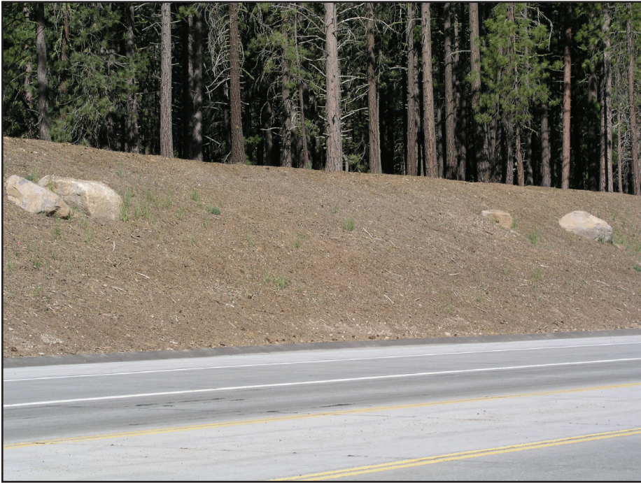
Figure 8a—Wood mulch on cutslope with vegetation starting.
