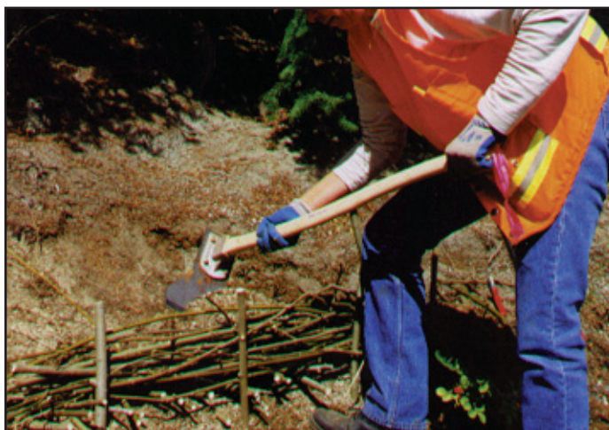
Figure 15—Brushlayer modified with willow fencing. (Lewis 2000)
