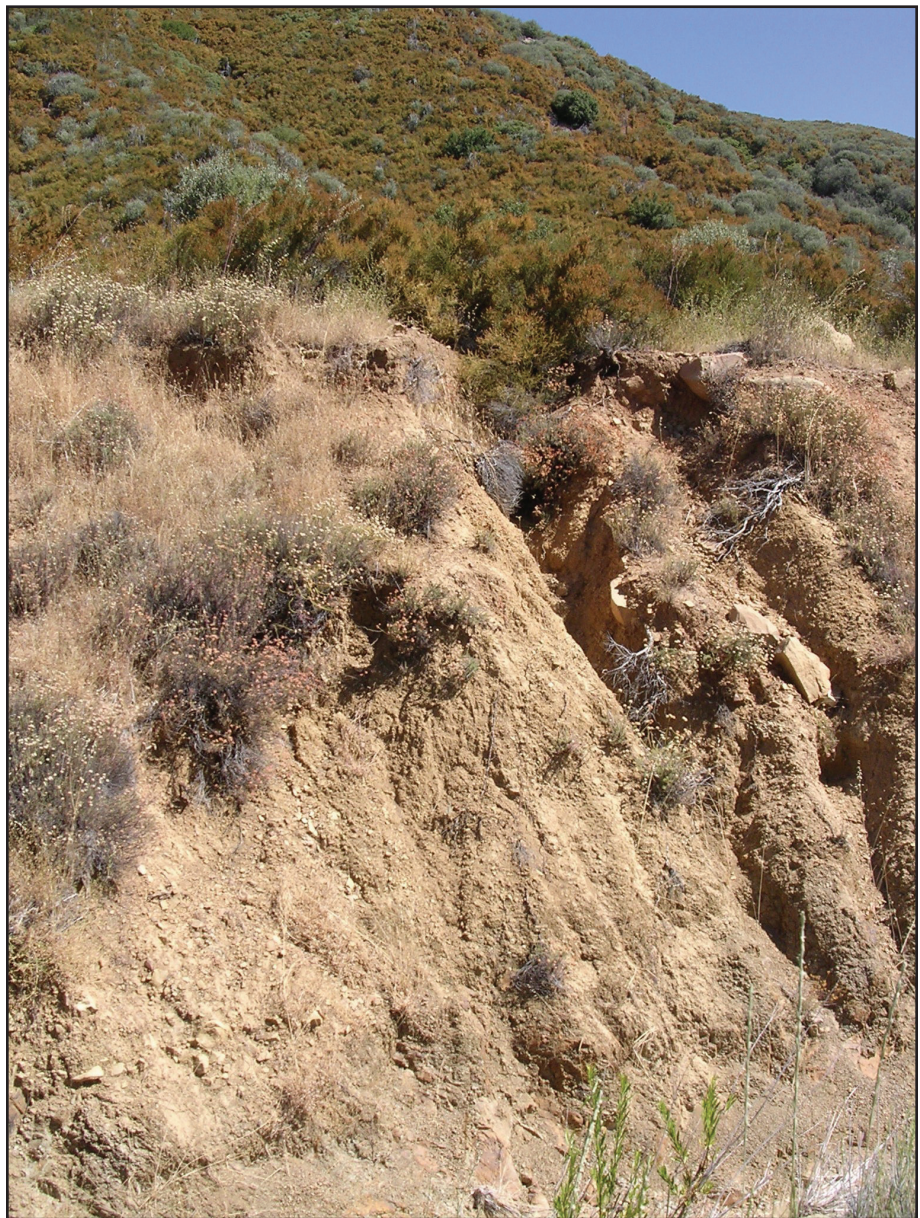
Figure 2—Interrill (sheet) erosion with rills and gullies forming.
