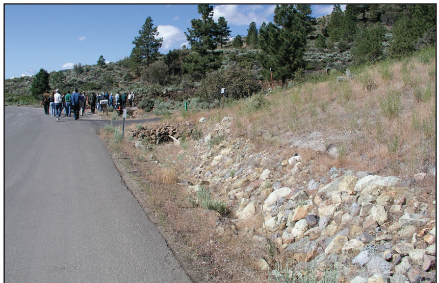
Figure 6—Relatively recent cutslope vegetated with native seeding.
