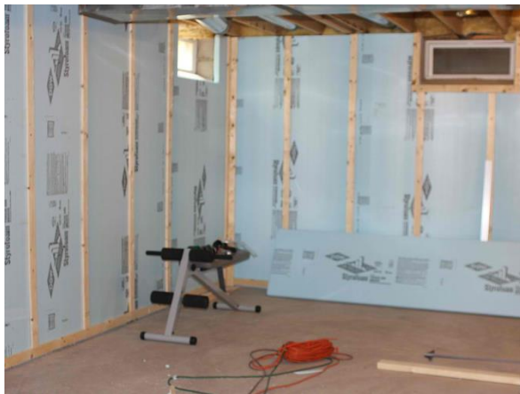
Interior insulation R-15 continuous
