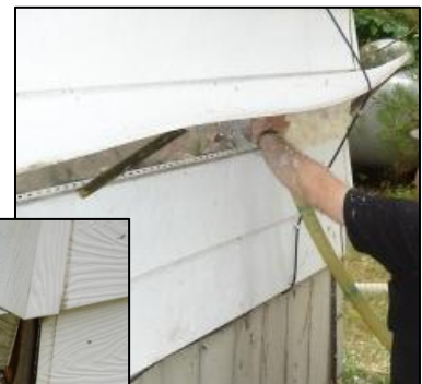
Blowing walls: Using a fill tube works well for most mobile home wall cavities.
