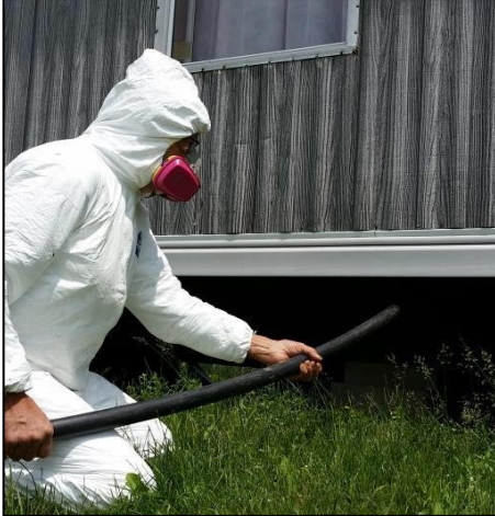
Fill tube inserted into belly hole.
