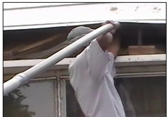
Roof-edge blowing: Use a rigid fill tube to blow insulation through the roof edge. This avoids making holes in the roof, though this process requires much care in refastening and re-sealing the roof edge.
