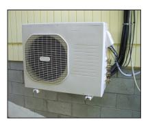
Outdoor unit with compressor and heat exchange coil
