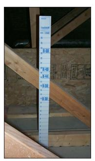
Figure G-1 Insulation depth marker
