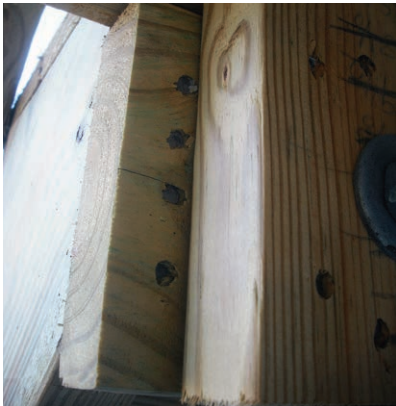
Figure 4. Nails driven through a dropped header into the end grain of a stringer (above left) have minimal resistance to withdrawal. Toenailed stringers are less susceptible to withdrawal, but the connection can still fail as the framing ages and is structurally compromised (above center). At a cost of a few dollars each for the connectors and recommended fasteners, the most cost-effective way to hang a stringer is with metal hardware. But this one (above right) has been installed incorrectly, since the stringer isn't fully bearing on the connector seat. Another red flag: drywall screws instead of approved connector fasteners.
