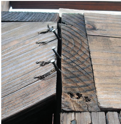
Figure 4. Nails driven through a dropped header into the end grain of a stringer (above left) have minimal resistance to withdrawal. Toenailed stringers are less susceptible to withdrawal, but the connection can still fail as the framing ages and is structurally compromised (above center). At a cost of a few dollars each for the connectors and recommended fasteners, the most cost-effective way to hang a stringer is with metal hardware. But this one (above right) has been installed incorrectly, since the stringer isn't fully bearing on the connector seat. Another red flag: drywall screws instead of approved connector fasteners.
