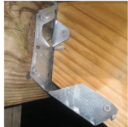
Figure 4. Nails driven through a dropped header into the end grain of a stringer (above left) have minimal resistance to withdrawal. Toenailed stringers are less susceptible to withdrawal, but the connection can still fail as the framing ages and is structurally compromised (above center). At a cost of a few dollars each for the connectors and recommended fasteners, the most cost-effective way to hang a stringer is with metal hardware. But this one (above right) has been installed incorrectly, since the stringer isn't fully bearing on the connector seat. Another red flag: drywall screws instead of approved connector fasteners.
