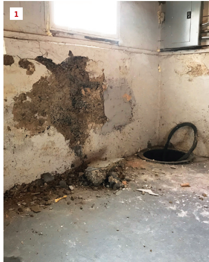
This area of the existing foundation was weak but still structurally sound (1). In their investigation, the crew discovered that there was no footing under the original foundation (2) and turned to an engineer for a solution.
