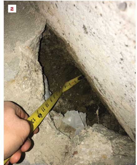
This area of the existing foundation was weak but still structurally sound (1). In their investigation, the crew discovered that there was no footing under the original foundation (2) and turned to an engineer for a solution.
