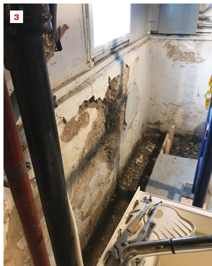
The crew cut the slab and dug a footing trench 1 foot wide and 1 foot deep (3). Under the wall, they dug 2-foot-wide voids 2 feet apart that would be filled with concrete as part of the new footing. A special tool bends rebar into the needed shapes (4).
