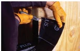
Make vertical relief cuts starting from corner of window sill upward. Roll firmly into place as necessary.
