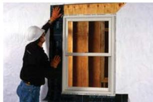
Unroll flashing by removing the release paper exposing the adhesive. Roll firmly into place as necessary.
