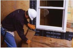
Unroll flashing and expose adhesive by removing the release paper. Roll firmly into place as necessary.
