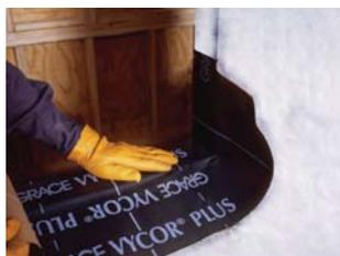
Apply flashing to window sill by removing half of the release paper and exposing the adhesive. Roll firmly into position.
