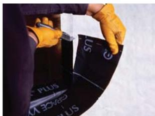
Make vertical relief cuts starting from corner of window sill upward. Roll firmly into place as necessary.
