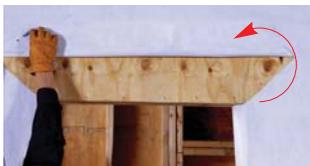
**Score and fold weather-resistive barrier above header. Temporarily secure to allow for flashing installation.**
