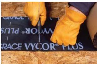
The length of the flashing should extend beyond the sill equal to the width of the jamb flashing (see Table I, page 8).
