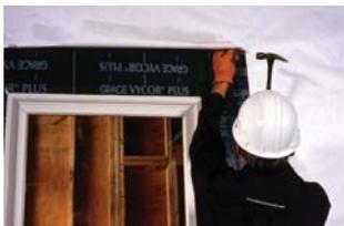
Mechanically fasten head flashing at top outermost corners, as necessary.
