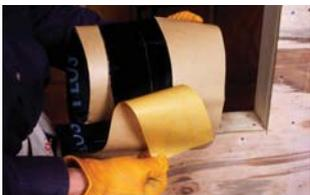
Split the release paper in half allowing for easy installation.
