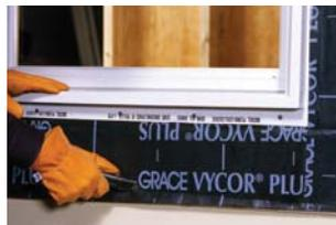
Trim excess flashing that hangs below the nailing flange.
