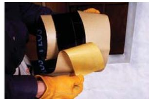
**Split the release paper in half allowing for easy installation.**
