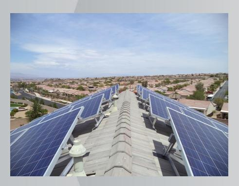
Supports for solar modules are to be installed to spread the dead load across as many roof framing members as needed, so that no point load exceeds 50 pounds.
