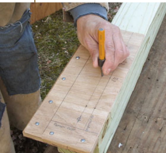
Figure 6. A site-built jig ensures accurate hole placement. The author marks the hole locations with a nail set.
